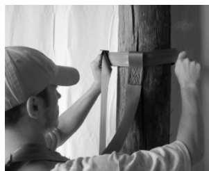
Figure 13 INSTALL BELT BELT AT OR ABOVE EYE LEVEL
