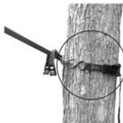
Figure 33 Secure Tree Brace Using Ratchet Strap
