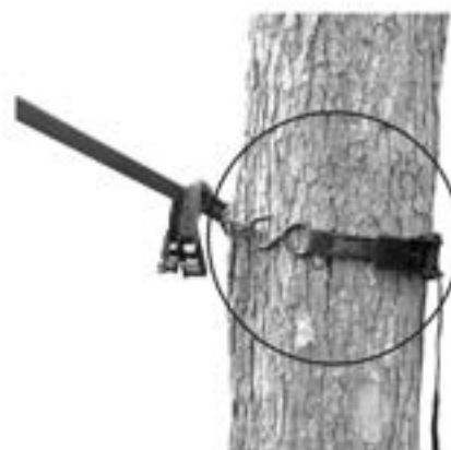
Figure 33 Secure Tree Brace Using Ratchet Strap
