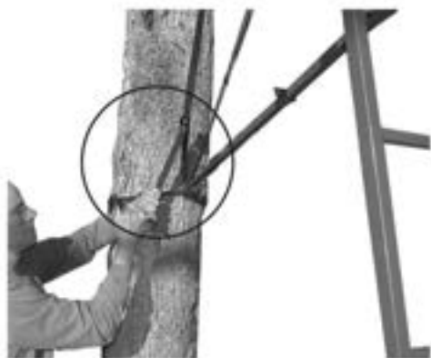
Figure 34 Stabilizer Straps Installed
